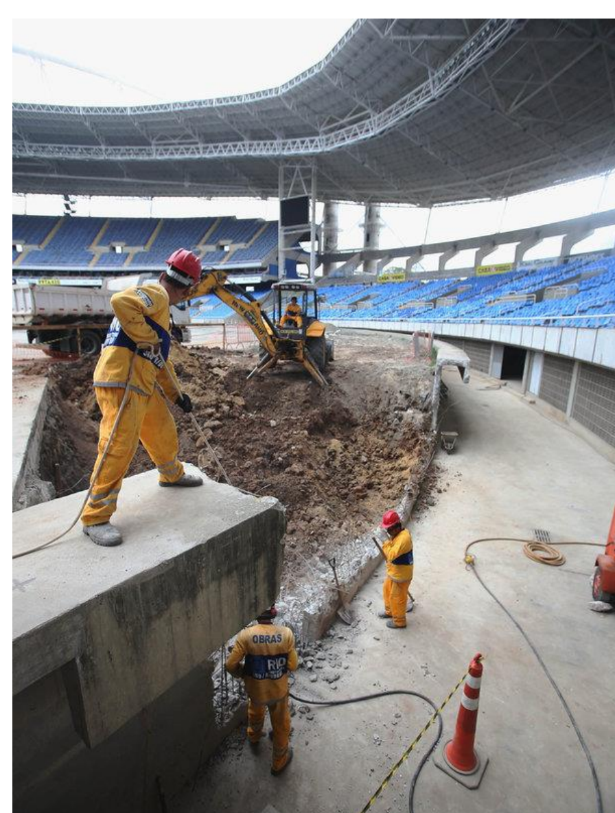
Stadium Construction by NPR
